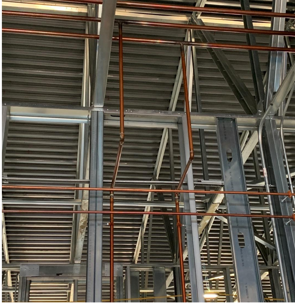
The above picture was taken looking west. The next picture is of the same room looking south.
